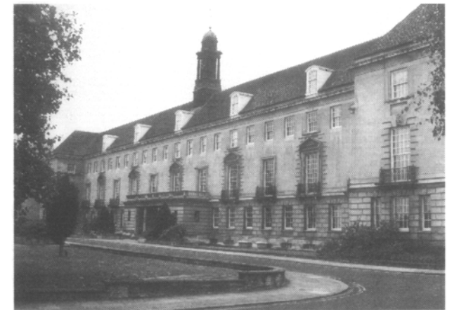
County Hall, Bythesea Road
