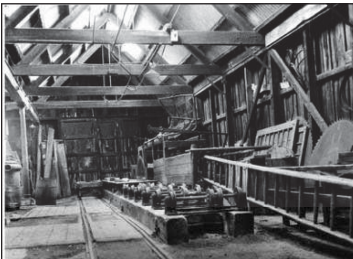
Sawmill. Note the railway to bring uncut tree trunks in from outside. Circular saw is at far end of the floor-mounted rollers, on the right.
