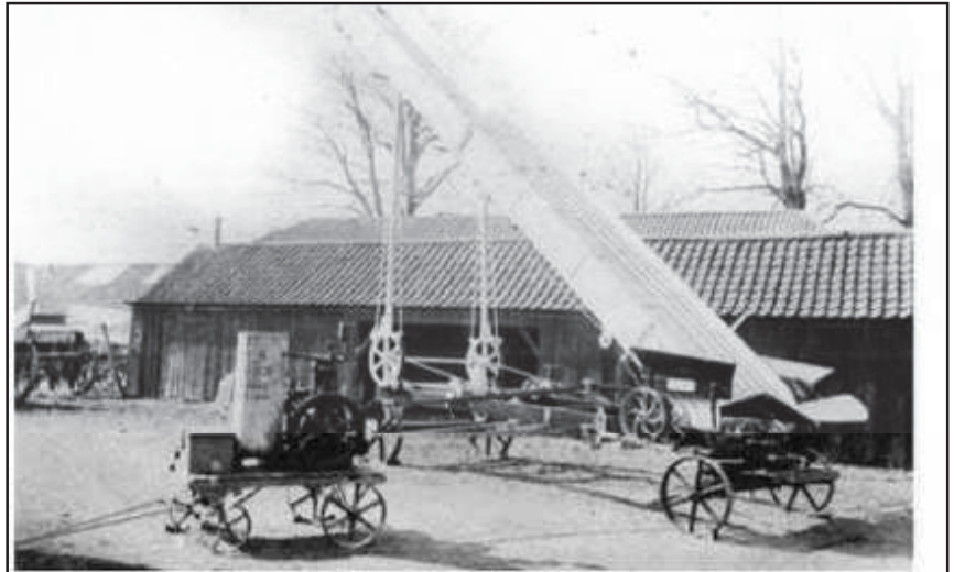
Reeves 'Advance' elevator, with troughs raised. Chains are driven by a Fairbanks Morse portable oil engine, through belt drives. The two-storey building in the distance houses the carpenters' shop (ground floor) and tinsmiths' shop above. Circa 1912
